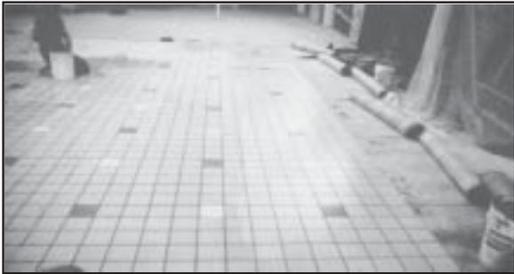
Installed between the bonding agent and the flooring, the sheeting isolates the tile to prevent cracking and ensures uniform thickness and quality. The 55-year-old Michigan-based Noble Company offers a lifetime guarantee on its NobleSeal TS.
