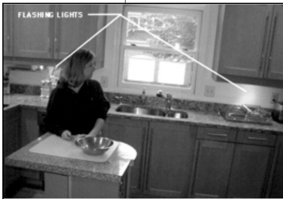
Flashing lights alert resident to the doorbell activation of the doorbell.
