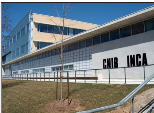
A large window wall provides ample natural light.
