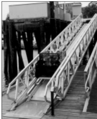
Other safety features include: self-leveling capability regardless of water level; an audible alarm that sounds when the car travels without a rider; mechanical and electrical interlocks on the door; and a key-reset thermal interlock to prevent travel in freezing temperatures.
