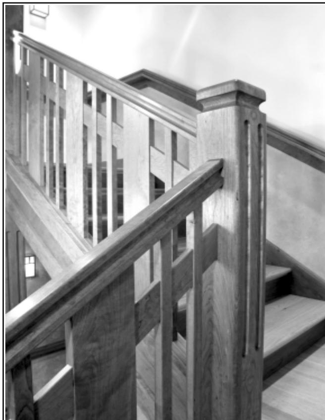
Alan Abrams, the designer who detailed much of the craftsman woodwork details in the house, developed a handrail section that allows opposition between the thumb and fingers, allowing a more secure grip.
