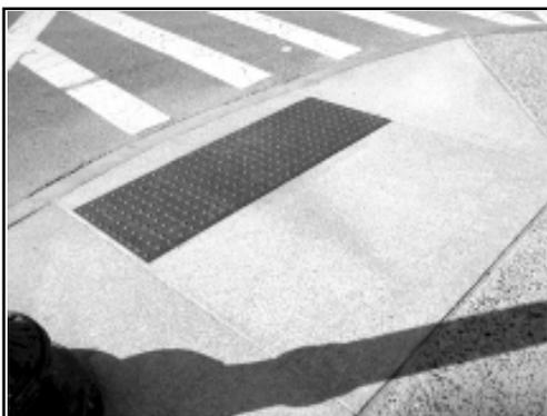
Curb Ramp 3 features granite construction common in Washington, DC.
