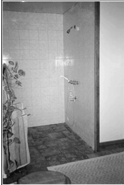
The curbless shower features water temperature and flow controls at 34 inches.
