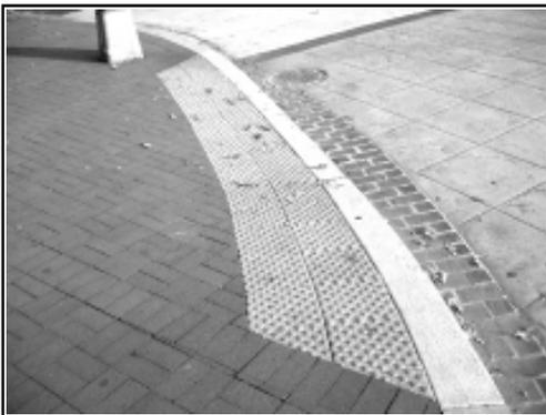
Curb Ramp 2 features integral detectable warnings.
