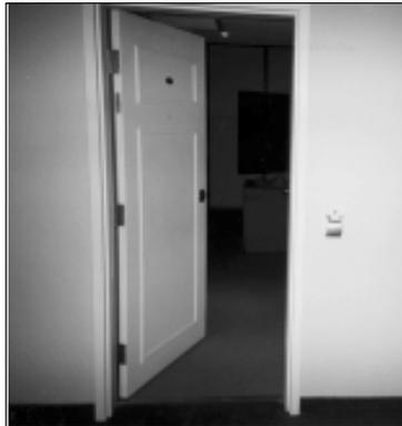
This system eliminated the need for maneuvering space at the door, and created an upscale amenity that impresses the most demanding of guests. There is no handle on the outside of the guestroom entry door. A swipe of the keycard both unlocks the door and activates the automatic opener, making it easy to roll your luggage or wheelchair directly into the room. To exit the room you can either push a button on the wall or operate the standard lever handle on the inside face of the door. ■
