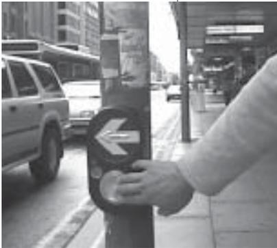
The Panich audible, vibro-tactile accessible pedestrian signal has a repeating locator tone that changes to a faster repetition rate during the “Walk” interval. The sound comes from the pedestrian button. The raised arrow points toward the crosswalk and also vibrates during the “Walk” interval.
