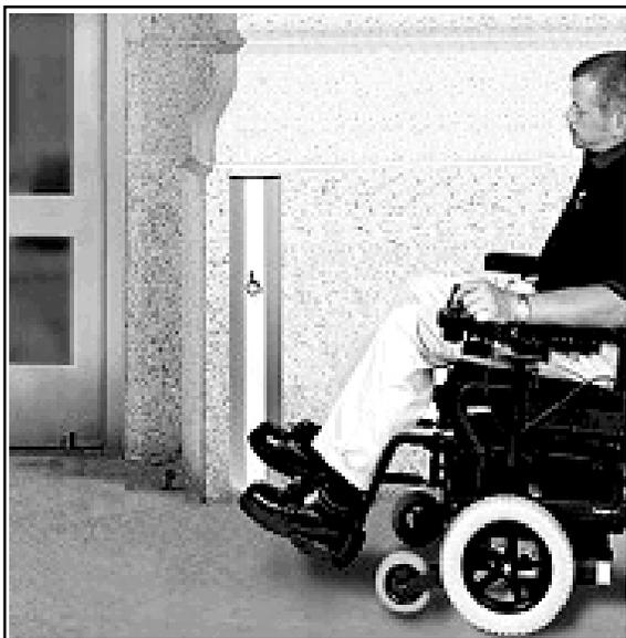
inch tall door operator switch serves people of all abilities by means of a tap at any point along its height.
