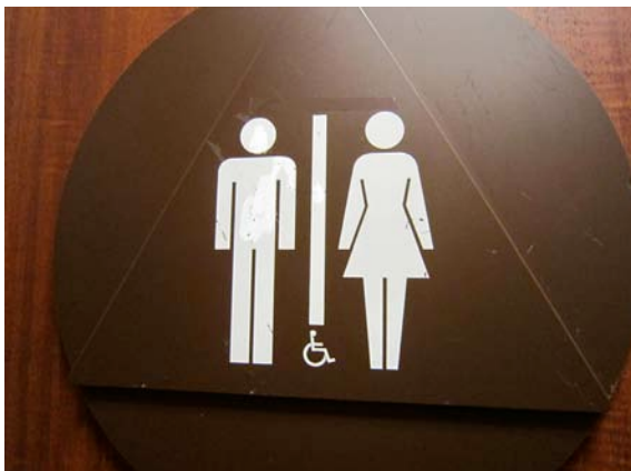
California accessibility code requires circular signs for women's restrooms, triangular signs for men's restrooms and a triangle on top of a circle for unisex restrooms. In this case, the purpose of the signs has been defeated by choosing the same brown shade for both signs.
