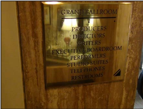
This sign's finish creates reflections and glare, making the sign extremely difficult to read.
